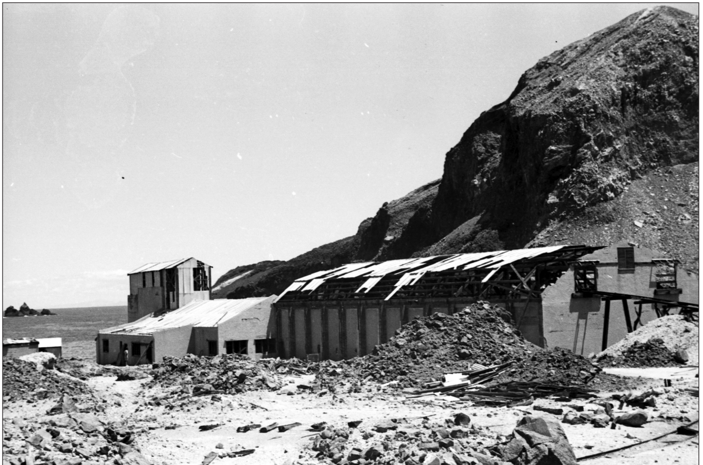
Figure 1. The abandoned sulphur factory on White Island, November 1949, where Wodzicki trapped and identified kiore. Photo by Kazimierz Wodzicki.
