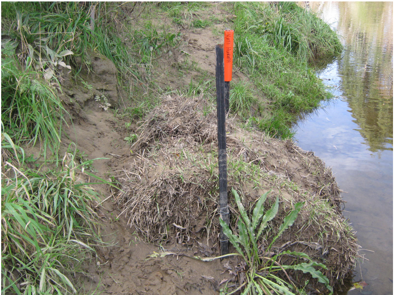
Figure 2. Straw bales in position at Orbell’s Crossing spawning site (R Clucas). Note the fines deposited on and around the bales following a fresh tide. Good drainage of the bales was required between spring tides to encourage spawning.
