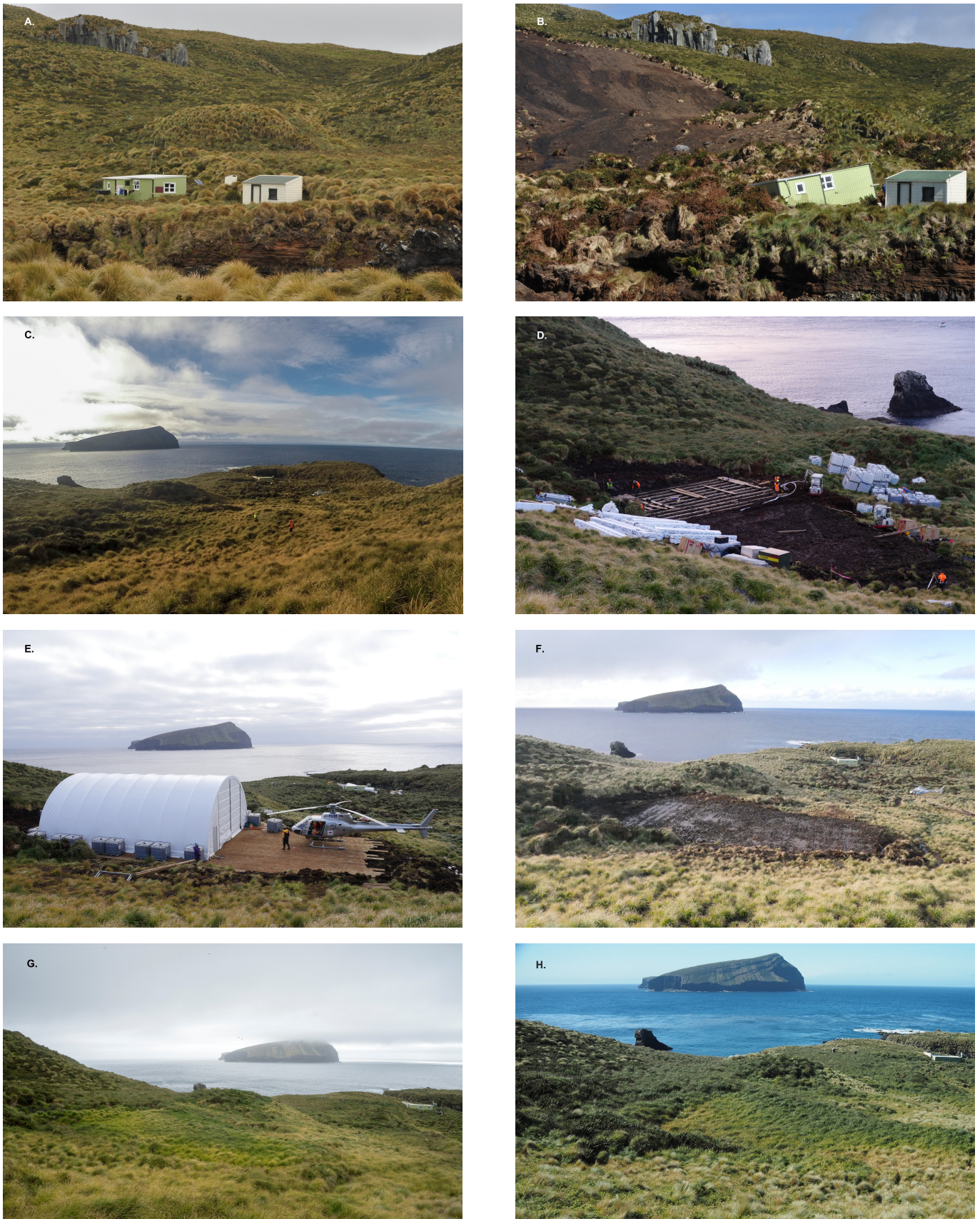
Figure 7. Vegetation disturbance and recovery at the temporary helicopter hangar site on Antipodes Island. Images shown in order: (A) field hut and historic castaway depot; (B) field hut and historic castaway depot post landslip January 2014; (C) hangar site pre-clearance 28 May 2016; (D) hangar site post-clearance and during construction; (E) hangar site with hangar completed 5 June 2016; (F) hangar site following removal of the hangar 3 August 2016; (G) hangar site with tussock cover 3 March 2018; (H) hangar site 5 February 2021 (Photos: A, B & H – KJW; C, D, E & F – SRH; and G – FSC).
