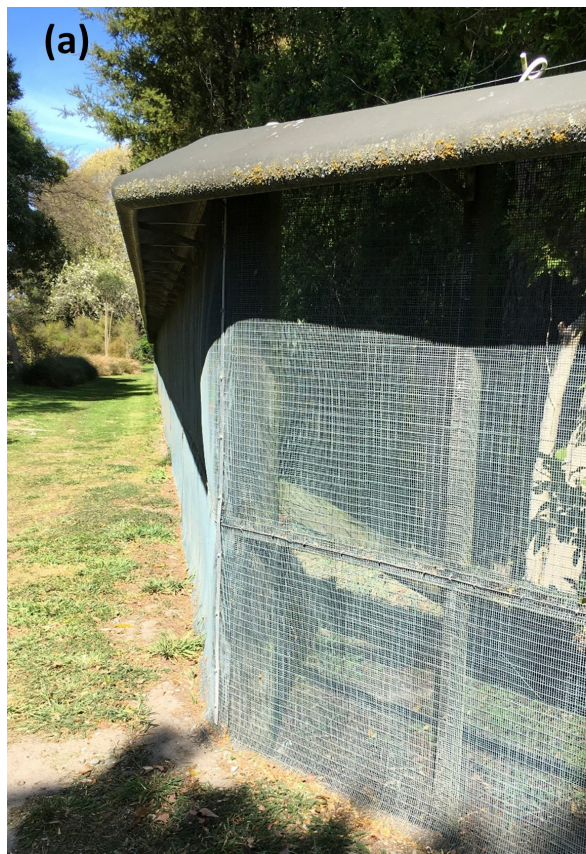
Figure 3. A fence constructed with a fine wire mesh, capped, and topped with an electric wire has been used at Riccarton Bush, Christchurch, to exclude invasive mammal predators such as brushtail possums, stoats and rats (a). Simpler fences constructed with a coarse wire mesh have been used in Te Urewera to exclude invasive mammal herbivores such as deer (b). Such fencing treatments are widely deployed for animal exclusion but often exclude non-target species, have been located subjectively, treat a small area, are subject to periodic breaches, and potentially influence ecosystem-level responses (e.g. seed production and litter fall).
